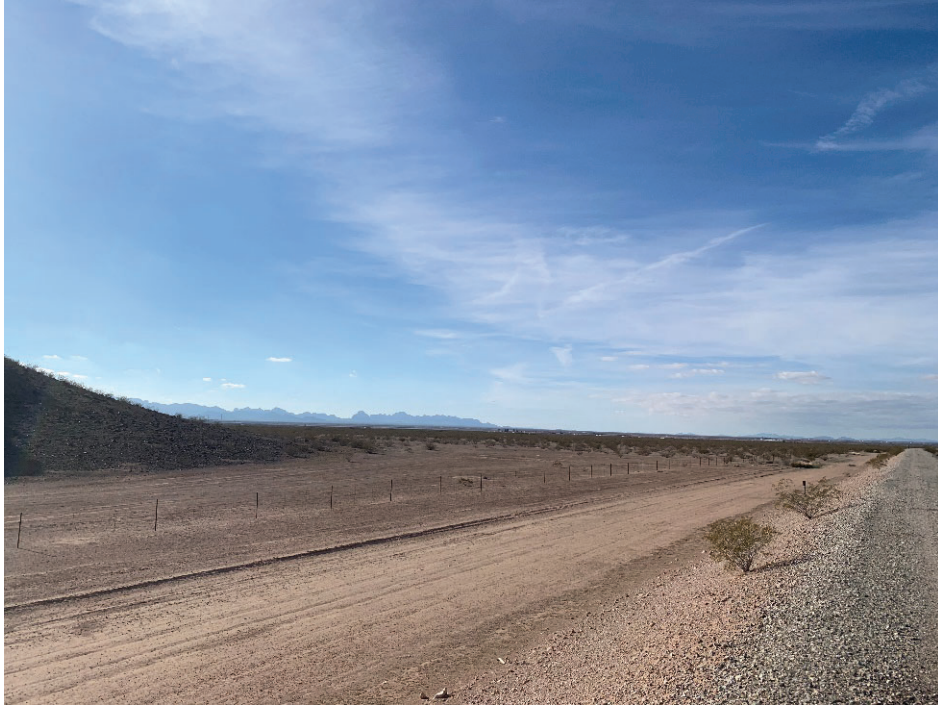
View from FCDMC Saddleback Flood Retarding Structure facing west towards projects limits
