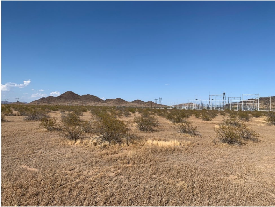
Photo 5. Photograph faces northeast. Delaney Substation is in the right of the photograph
