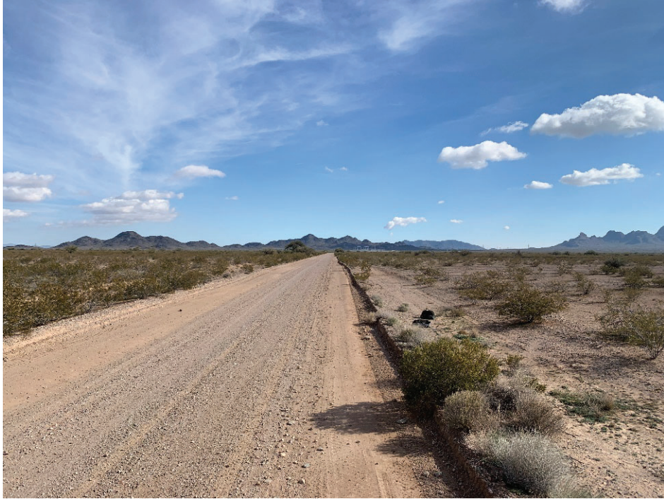
View along Salome highway in center of project area facing southeast
