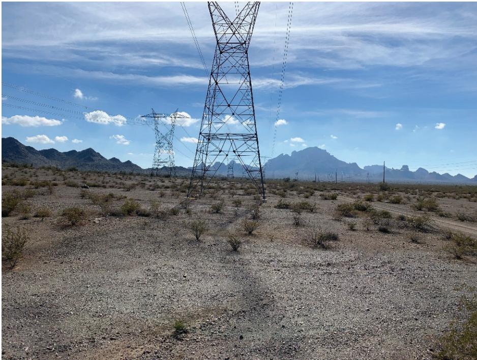
View of project area from Indian School Road facing south along existing transmission line
